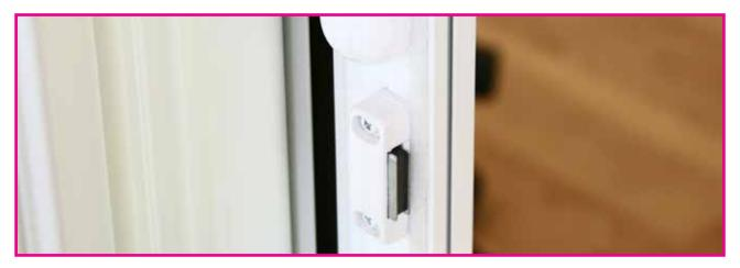
Close the screen door so you can see where to mount the metal strike plate. Mark out two holes and screw fast the strike plate, se below.
