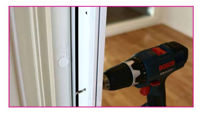
Use the 4 cm screws to install the handles. Don't forget to cover the screws with the thin plastic covers.
