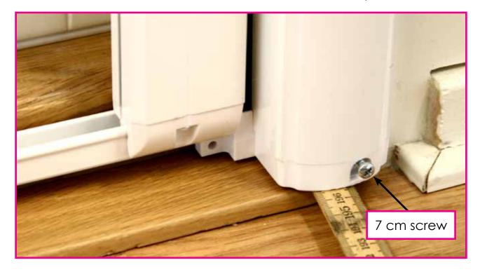
Slide in the bottom rail through the pullbar so the pre drilled hole lines up as you practiced earlier on the floor. It's important that the end of the rail with the diagonal cut is connected to the housing. Next, screw in the two 2 cm screws as per below, but only half way. Remember to make sure that the bottom rail and housing are at 90 degrees.
